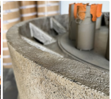
Fig. 2. Manual cleaning of the inside of the runner hub — hub cover prior to overhaul
