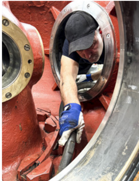
Fig. 2. Manual cleaning of the inside of the runner hub — hub cover prior to overhaul
