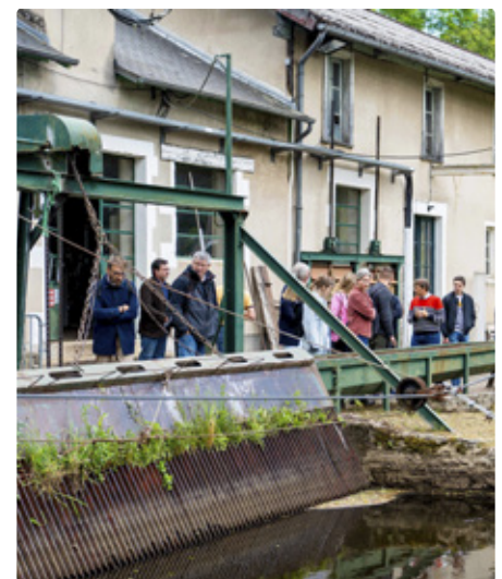
Fig. 2. Beaufort Mill – water intake for hydro units – view from the high-level reservoir
