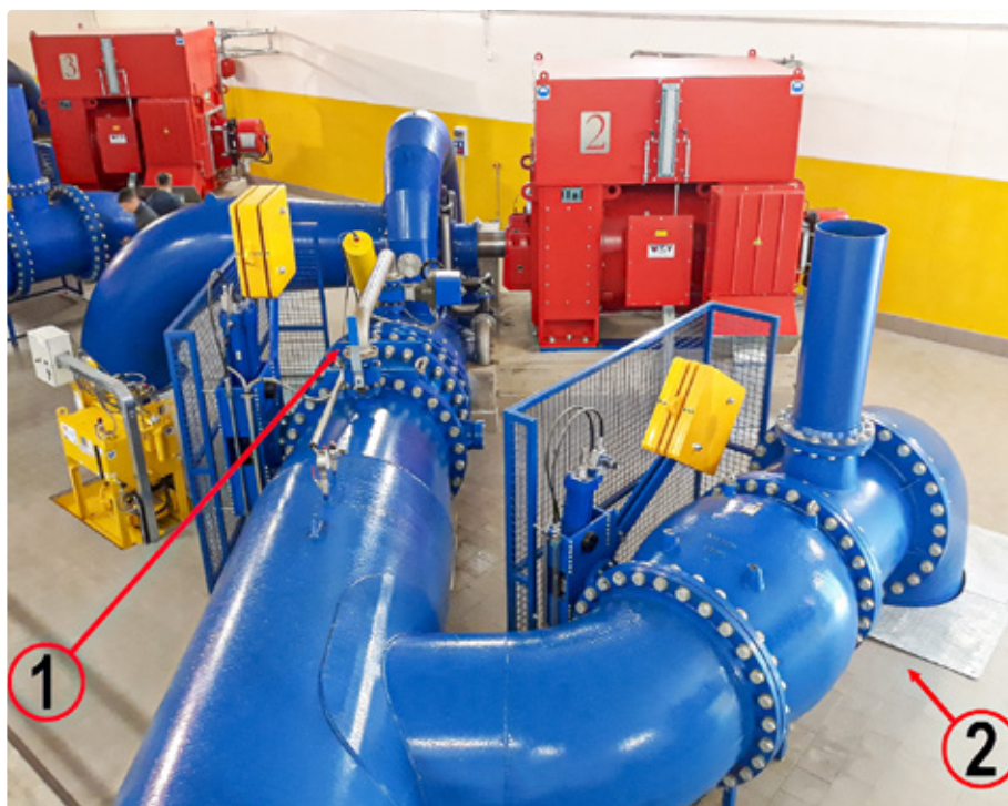
Fig. 9. An example of the implementation of a hydropower plant using T.I.S. fittings: 1. Double eccentric throttle with hydraulic cylinder and counterweight, together with mounting insert, 2. Needle valve with hydraulic cylinder and counterweight, together with an aeration device
