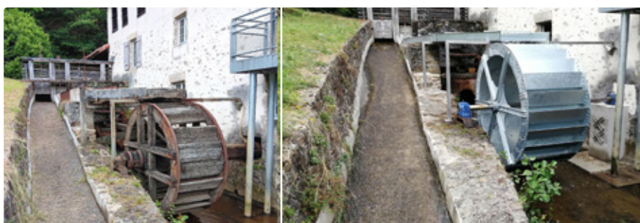
Fig. 5. The ancient wooden wheel recently replaced by a modern metal wheel
