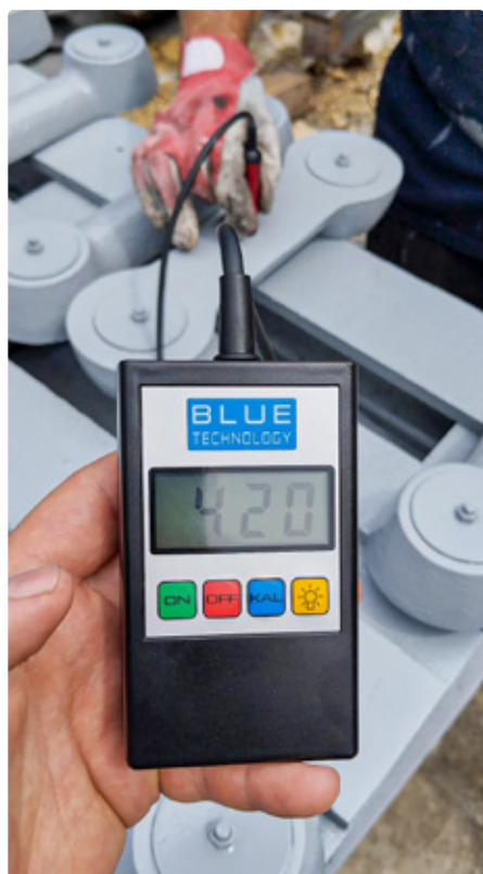
Fig. 12. Measuring the anti-corrosion coating during the coating application process
