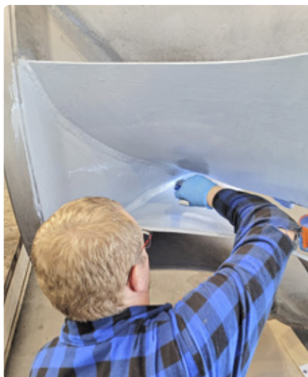
Fig. 5. Application of Belzona® 1341 coating
