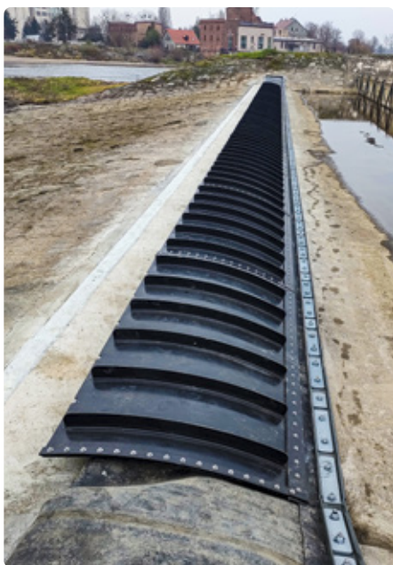
Fig. 3. Pneumatic movable weir with PE-HD flaps (Brzeg, the Oder River, 2022)
