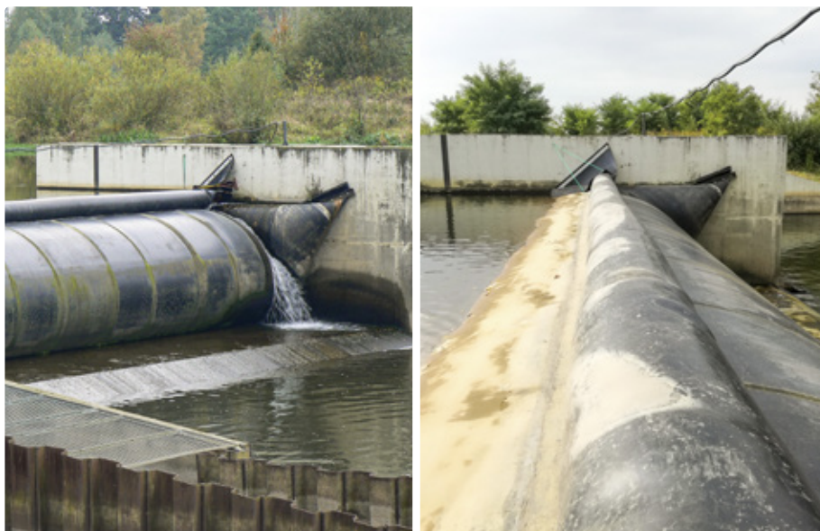
Fig. 2. Cascade weir (SHP Leszno Dolne, the Bóbr River 2018)
