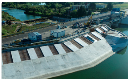
Photo. Rebuilding of reinforced concrete upstream slope
