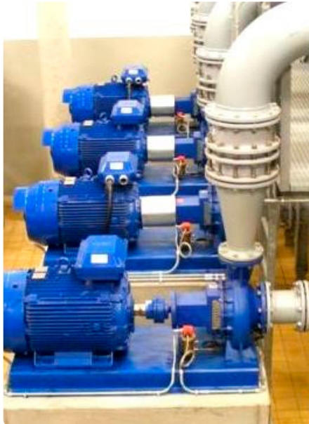
Fig. 5. Pump turbines in parallel arrangement
