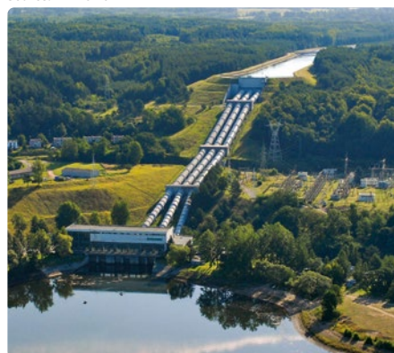
Fig. 3. The view of the power plant Żydowo, pipelines, and open channel
