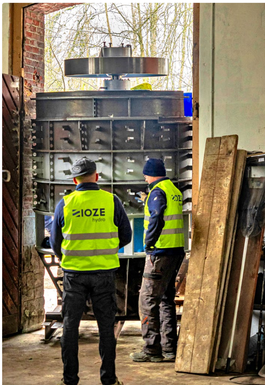
Photo: Bringing the turbines inside the watermill
