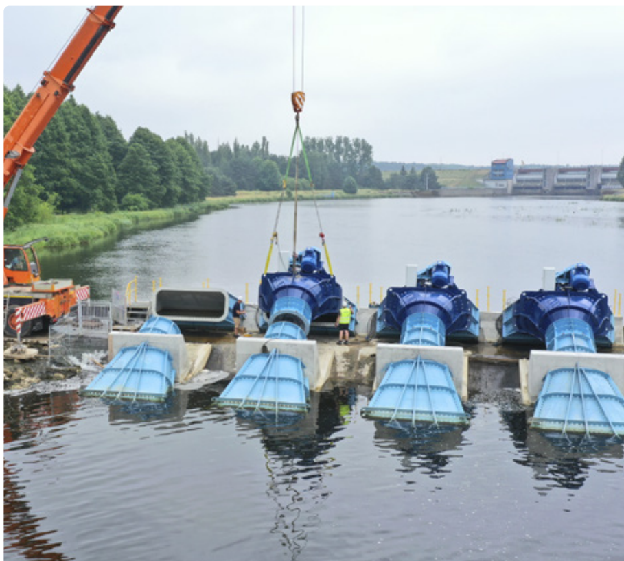
Photo. Assembly of siphon turbines
