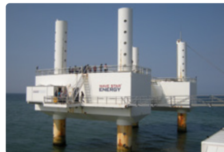
Photo 1. Wave Star wave energy converter prototype. Designed to use the same foundations as wind turbine
