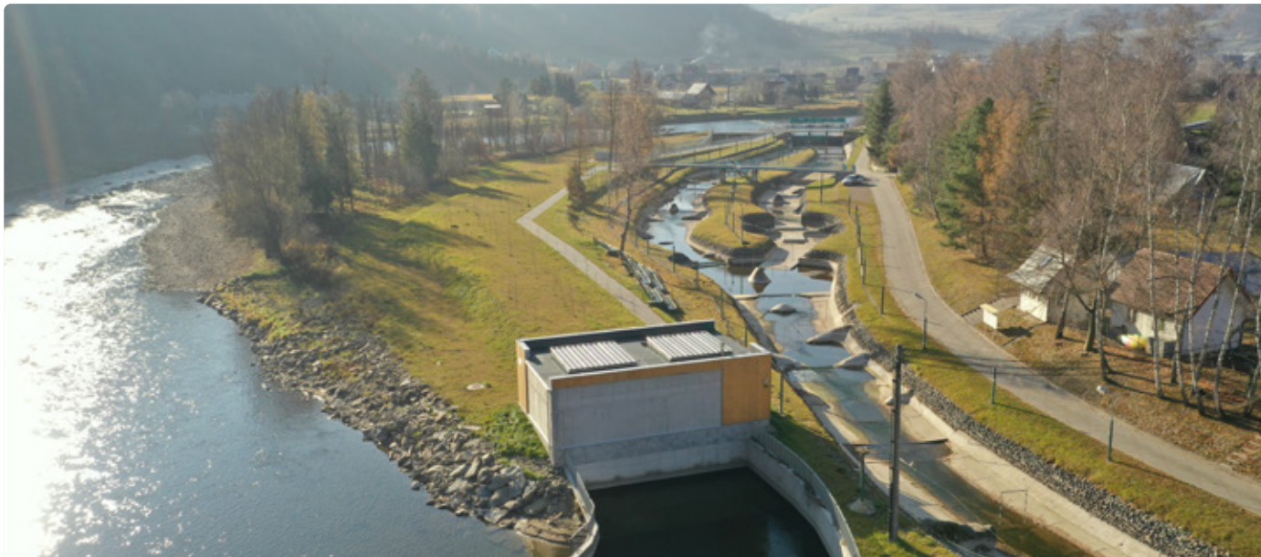
Photo. SHP Zabrzeż, Poland – by using the topography of the area in an appropriate way, the hydropower plant does not require the use of typical damming, thanks to which the river has retained its natural character and enables full fish migration.
