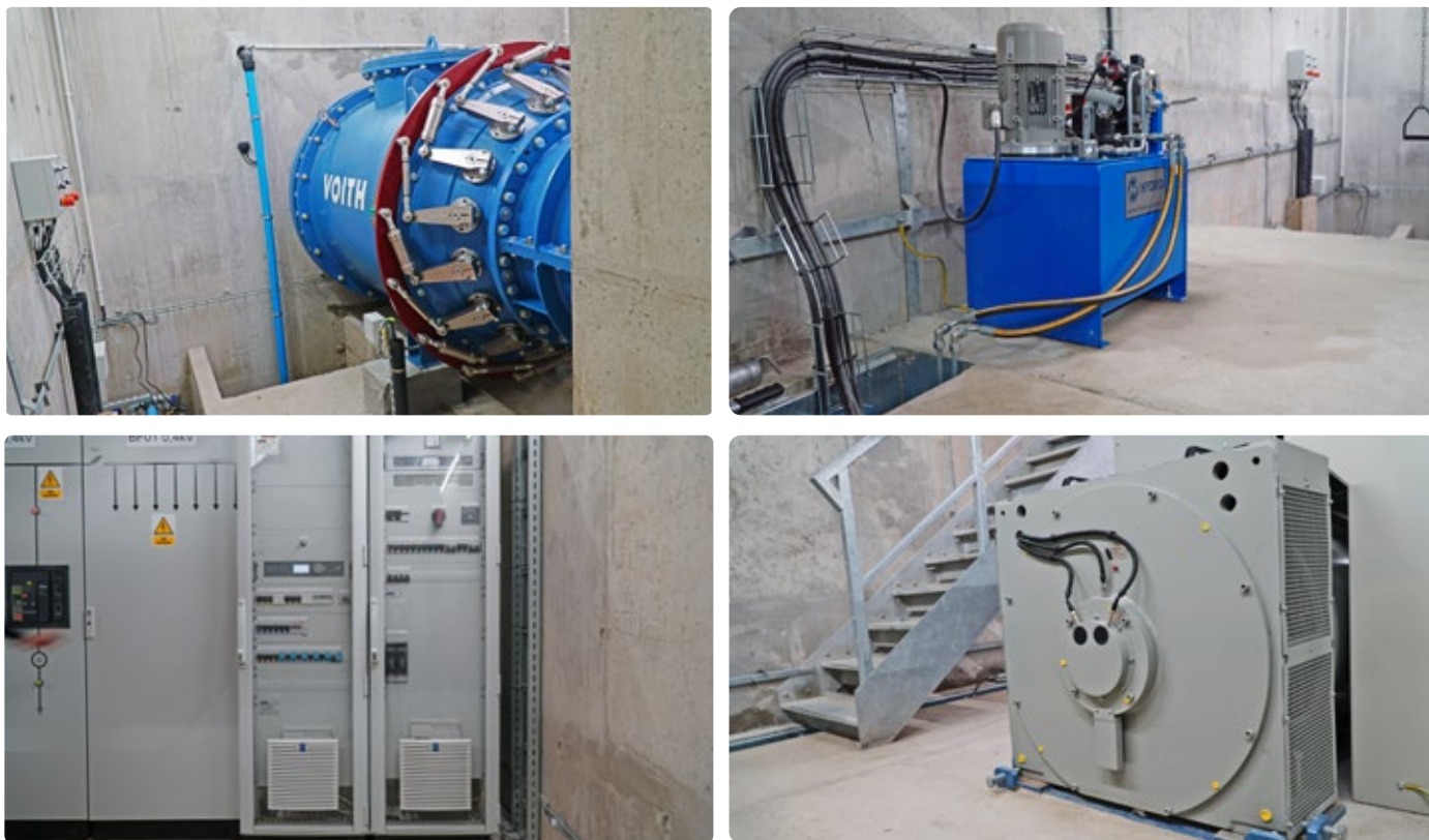
Photo 3. Key elements of the SHP equipment: water turbine, hydraulic power pack, electrical cabinets/turbine automation, synchronous generator
