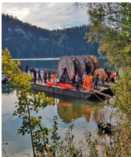
Photo 1. Laying a cable at the bottom of the Czorsztyn Lake
