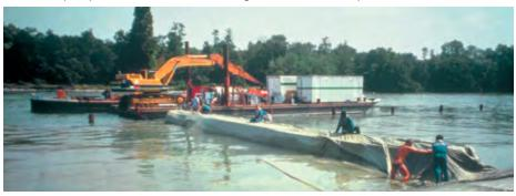
Fig. 9. Dychowski Canal, dragging an Incomat® panel from one bank to the other on support cables, 2018, photo: HZ-Bud.
