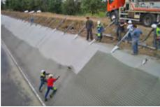
Fig. 7. Mittlere-Isar-Kanal, installation and concreting of the Incomat® Standard, bottom panel being lowered from the ramp, rolls of slope mats can be seen on both sides, *photo: Huesker.*
