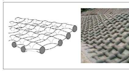
Fig. 6. Canal de la Gentile, (left) mats laid and top anchored, (right) sequential concrete filling, Incomat® Standard 1999–2000, photo: Huesker.
