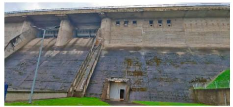
a length of 174 m and there were 70 thousand cubic meters of concrete expended on its construction. The object is made with 14 independent dilated concrete sections that are sealed at dilations with PVC tape. Sections number 7 and 8 are longer than the remaining ones (they are 15 m long, the rest are 12 m) and serve overflow protection and drainage functions.
