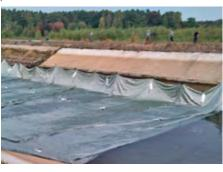
Fig. 10. Dychowski Canal, final phase of concrete pumping for part of the Incomat® Standard panel, 2018, photo: Inora.
