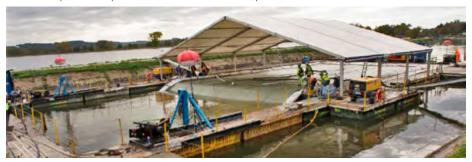
Fig. 8. Canal de Jonage, Installation of Incomat® Standard panel from a pontoon, together with the application of anchor loops to piles to stabilise the mats in flowing water conditions 1994, photo: Huesker.
