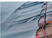
Fig. 11. Dychowski Canal, the left photo shows the concrete filled mattress before final treatment and the right photo shows the concrete mattress after the top flange has been cut off by approximately 1.0 m, [10].
