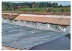
Fig. 10. Dychowski Canal, final phase of concrete pumping for part of the Incomat® Standard panel, 2018, *photo: Inora.*
