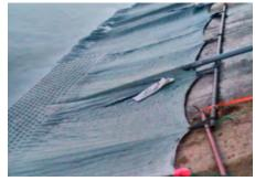
Fig. 11. Dychowski Canal, the left photo shows the concrete filled mattress before final treatment and the right photo shows the concrete mattress after the top flange has been cut off by approximately 1.0 m, [10].
