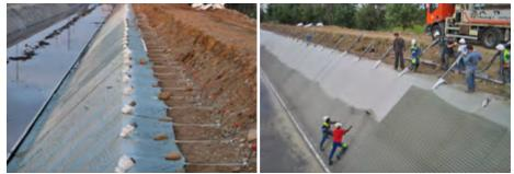
Fig. 7. Mittlere-Isar-Kanal, installation and concreting of the Incomat® Standard, bottom panel being lowered from the ramp, rolls of slope mats can be seen on both sides, *photo: Huesker*.
