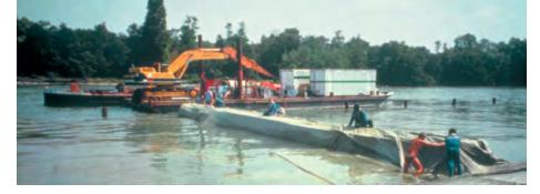
Fig. 9. Dychowski Canal, dragging an Incomat® panel from one bank to the other on support cables, 2018, *photo: HZ-Bud.*
